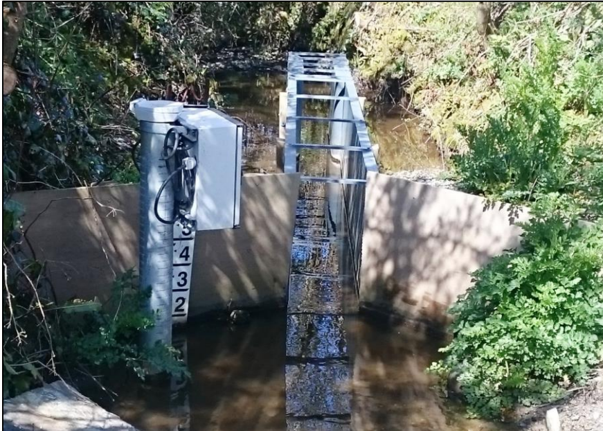
Figure B7/01-4-3 Flume and stage board at Location A
