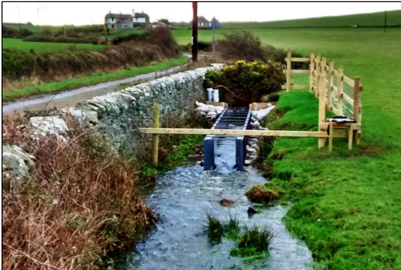
Figure B7/01-4-7 Flume and stage board at Location B
